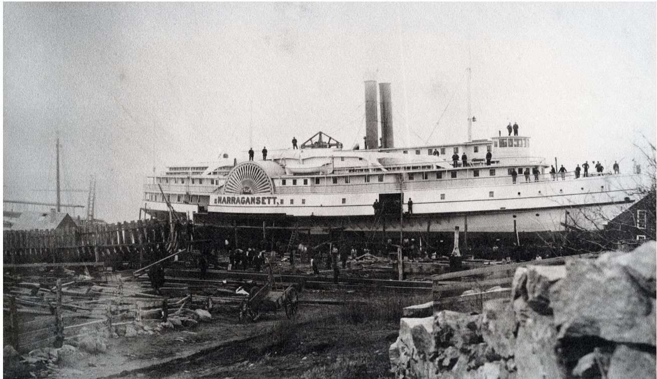
Photograph of the steamer Narragansett of the Providence & Stonington Steamship Co. on Palmer Marine R.R., Noank, being repaired after collision with the steamship Stonington . NHS1976.010, gift of Robert Palmer.
